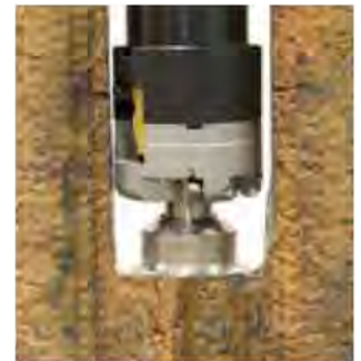
Remove membrane and overlay/cladding from between tubes
